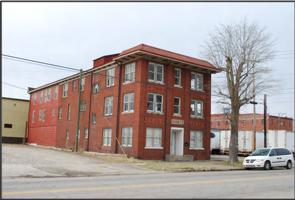
Figure 23. East and façade (north) elevations of the Barnett Hospital and Nursing School, looking to the southwest.
