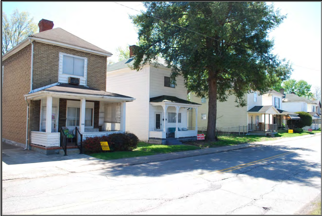
Figure 41. Dwellings along the south side of Ninth Avenue near Fifteenth Street, looking to the southwest.
