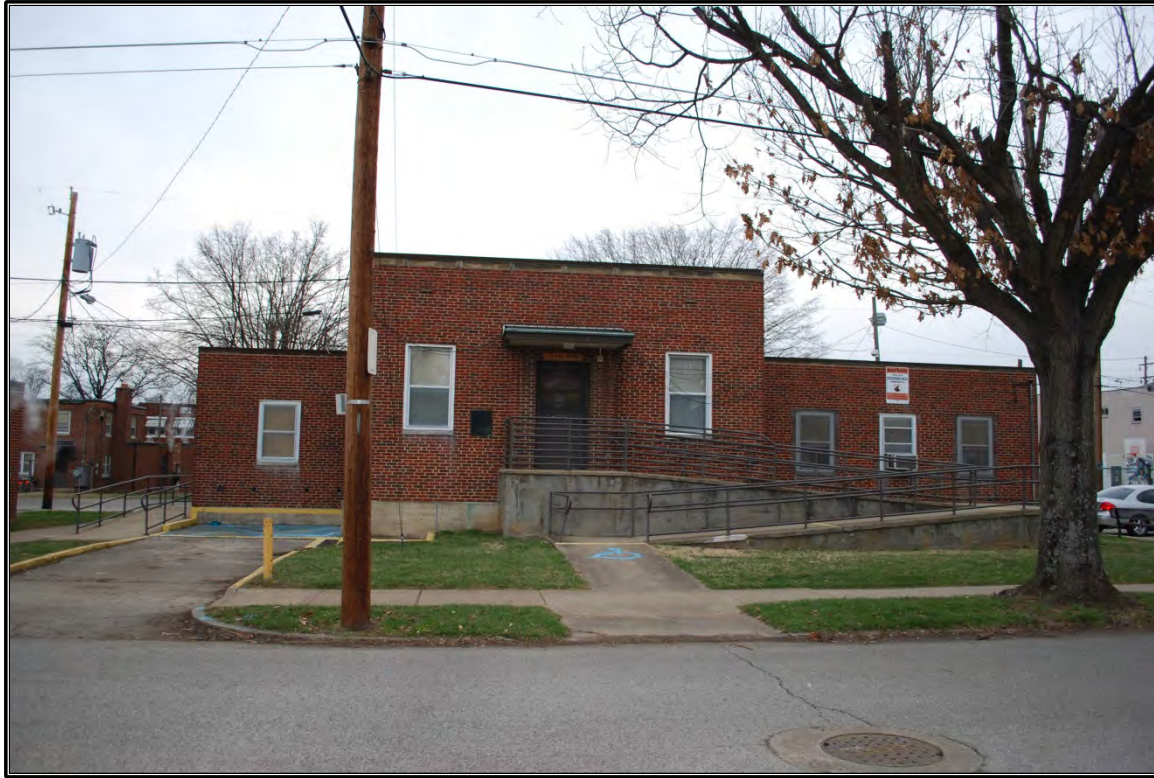
Figure 34. Façade (south) elevation of the Community Center building associated with Washington Square along Artisan Avenue, looking to the north.
