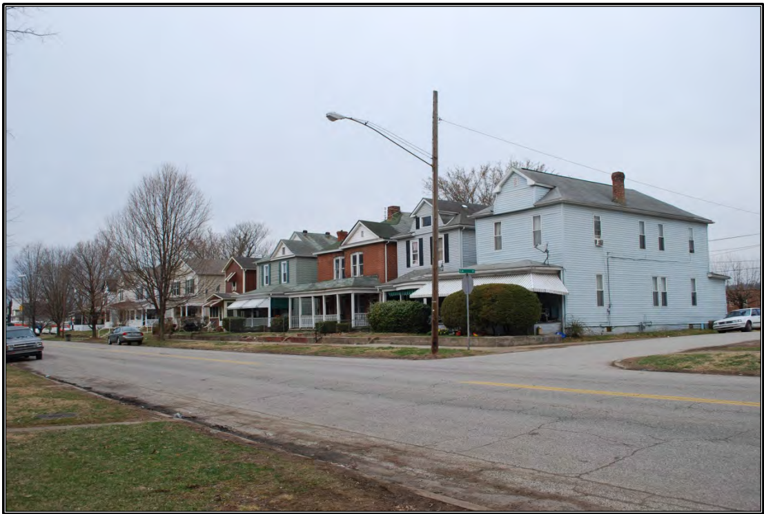
Figure 46. Residences along the north side of Ninth Avenue near the Sixteenth Street Baptist Church, looking to the northwest.
