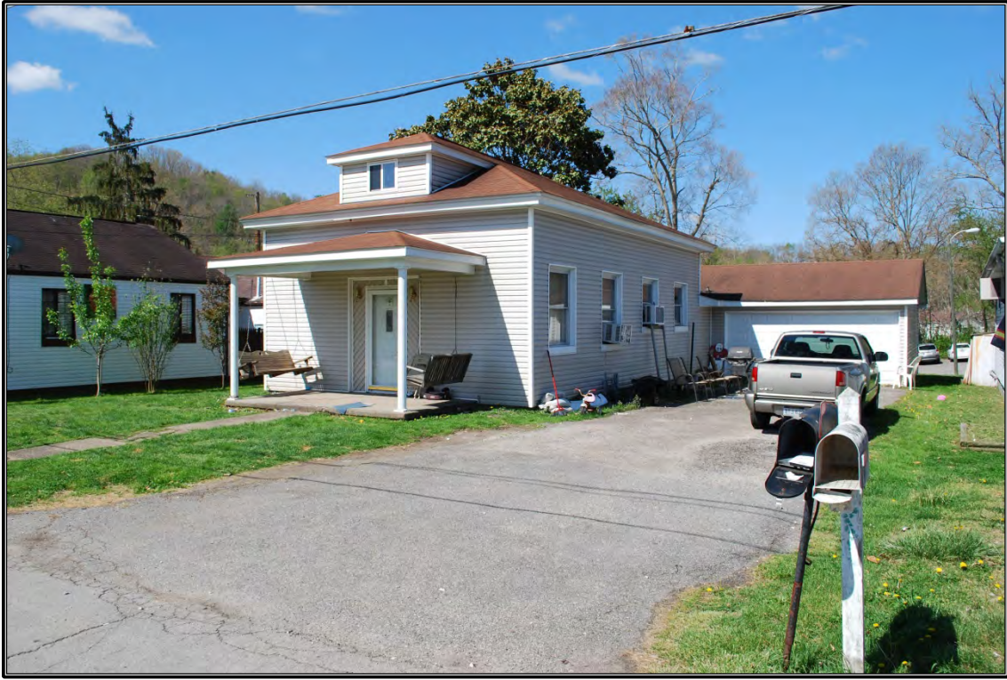
Figure 16. Façade (east) and north elevations of the former Barboursville Colored School, looking to the southwest.
