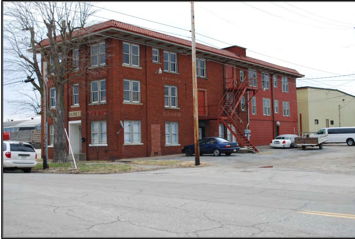
Figure 25. Façade (north) and west elevations of the Barnett Hospital and Nursing School, looking to the southeast.
