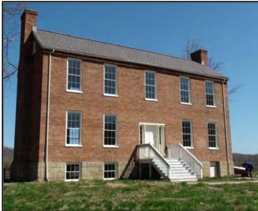
Figure 20. West and rear (south) elevations of the Albert Gallatin Jenkins house looking to the northeast (courtesy of the U. S. Army Corps of Engineers). 61
