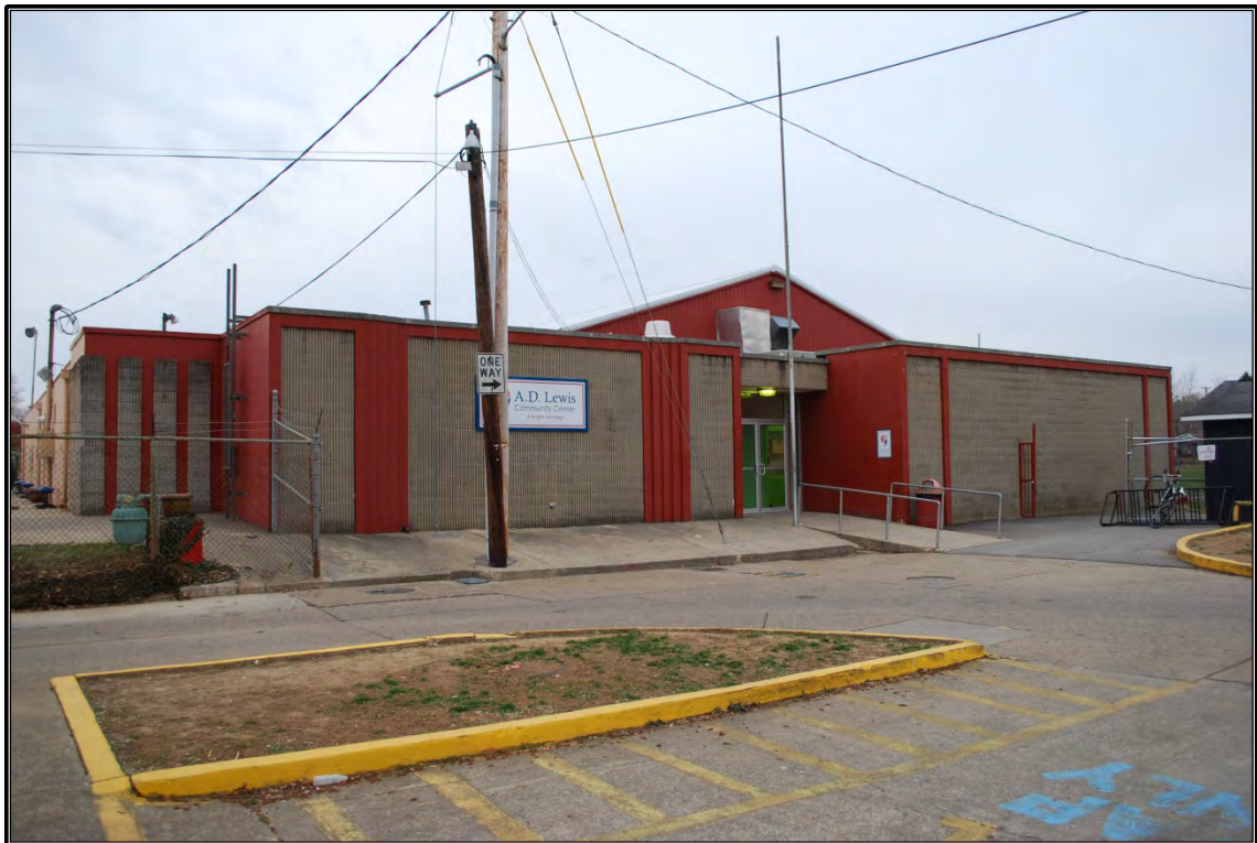
Figure 58. East and façade (north) elevations of the A. D. Lewis Community Center, looking to the south-southwest.
