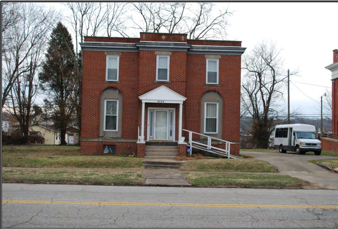
Figure 44. Façade (north) elevation of the Sixteenth Street Baptist Church's parsonage, looking to the south.
