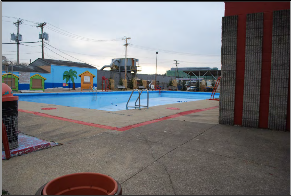
Figure 57. Overview of the swimming pool area, looking to the southeast.
