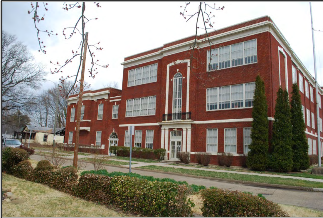
Figure 54. West and façade (south) elevations showing the side entrance to the main block of the school and the original gymnasium to the rear of the main block, looking to the east-northeast.
