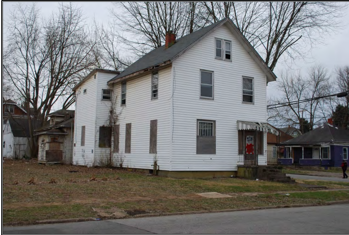
Figure 65. East and façade (north) elevations of the Memphis Tennessee Garrison residence, looking to the southwest.
